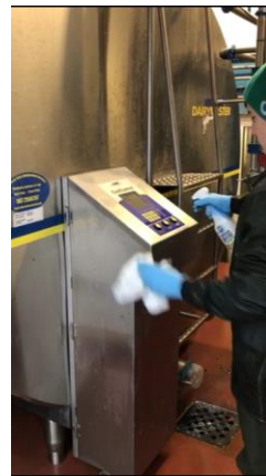
Clean control switches of bulk tank
